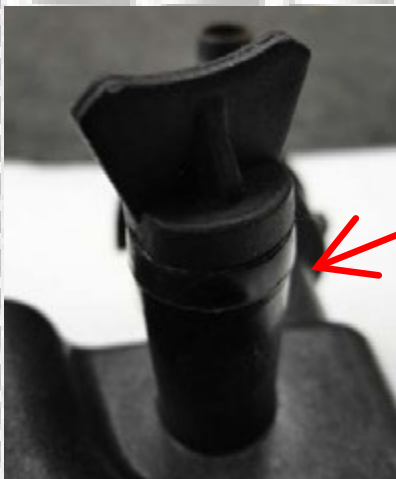
SPECTRA HEATER RETURN LINE WITH RUBBER CAP AND CLAMP (MAY REQUIRE REPLACEMENT EVERY 1-2 YEARS)
