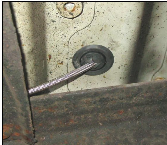
Figure 12 Floor access hole
