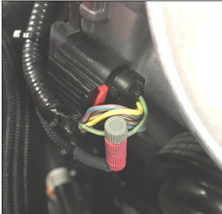
Figure 19 – TPS Signal Wires Connection
