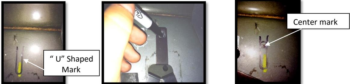
**Step 6:** Remove clip. Use a 1/2” drill bit and drill out the center mark. Slide the 3/8 clip back into position so the threaded part is aligned with the hole.
