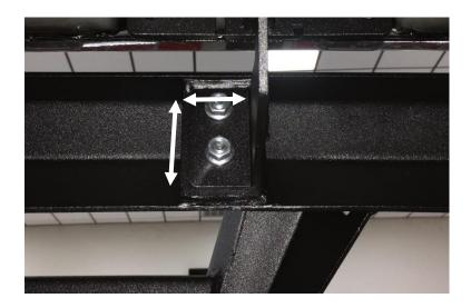
**Step. 9:** After finial positioning, completely tighten all (x6)  $\frac{1}{2}$ " -20 x  $\frac{3}{4}$ " in the pinch weld attachment.
