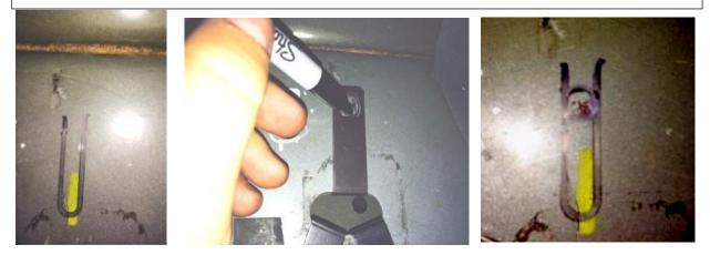
**Step 8:** Remove clip. Use a <sup>1</sup>/<sub>2</sub>" drill bit and drill out the center mark. Slide the 3/8 clip back into position so the threaded part is aligned with the hole.
