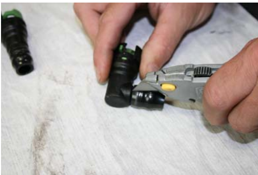
STEP 14 REMOVE REMAINING TUBE FROM FITTINGS
