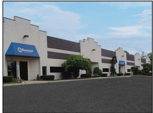
European Sales Office and Warehouse
