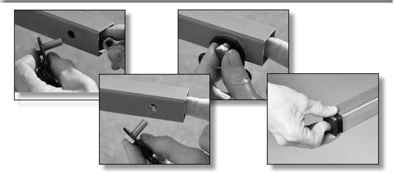
17. Align the bolt to the nut inside the cross bar and hand tighten. To secure fully, use a 9/16" wrench inside the cross bar to capture the nut inside. A 9/16" socket is used on the bolt head. Complete the cross bars with the new end caps. Repeat for remaining D-rings and end caps.
