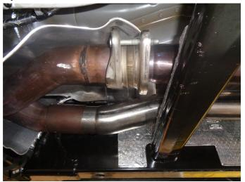
**Step 4.** Begin the installation by slipping the inlet of the P/S Inlet Pipe Assembly into the OEM band clamp. Engage the welded hanger to the rubber insulator. Next bolt the D/S Inlet Pipe assembly to the OEM flange junction using the supplied nuts. All clamps and fasteners are to remain loose until final installation.
