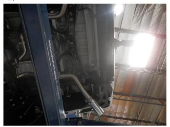
**Step 4.** Attach the Tail Pipes to the system using the supplied 2.50" clamps. Install the tips using a similar fashion with the supplied 2.75" clamps.
