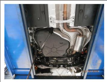
**Step 3.** Begin installing the new system by inserting the inlet of the Resonator Assembly into the clamp at the outlet of the OEM exhaust and fitting the hangers into the rubber insulators. Leave clamp loose for final adjustment.
