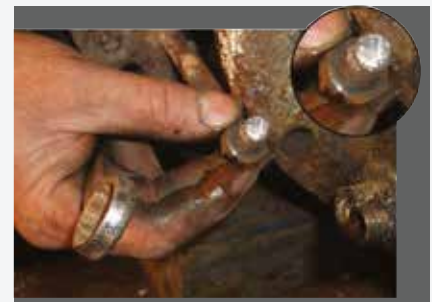
...which can lead to broken bolts.
