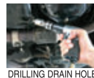
DRILLING DRAIN HOLE
