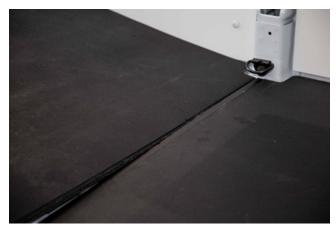
5. Join the h-track (rail) joint to the outerfacing edge of the second floor piece. Use a rubber mallet to firmly secure it to the floor piece.
