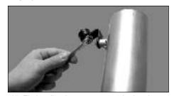
15. Fit the vibration mount on to the bracket using an M6 nylock nut & washer supplied.
