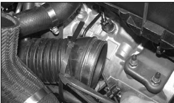
14. Using a pair of dykes, cut the clip tie that secures the vent hoses to the intake tube.
