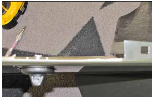
53. Using a cut-off wheel or similar tool, cut along the lines marked with the template and remove that section of the fender. Be sure to remove any remaining burrs with a file or deburring tool. NOTE: After cutting it is recommended using paint to cover the exposed metal to prevent rusting of the fender.
