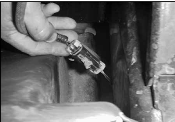
32. Detach the courtesy lamp wiring harness from the lower radiator cover and disconnect air temp sensor at the right bottom corner of radiator cover.
