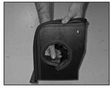
23. Install the provided edge trim into the hole of the heat shield as shown.
