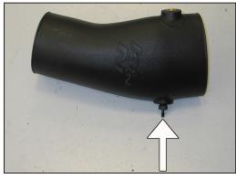
17. Install the provided 3/16" vacuum fitting into the K&N® intake tube as shown.
