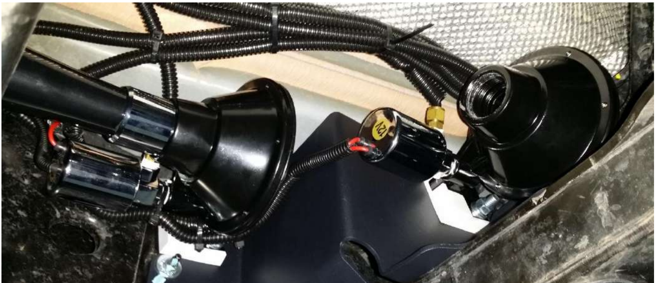
Figure 26 Horn Assembly Installed w/ Wiring and Air Lines
