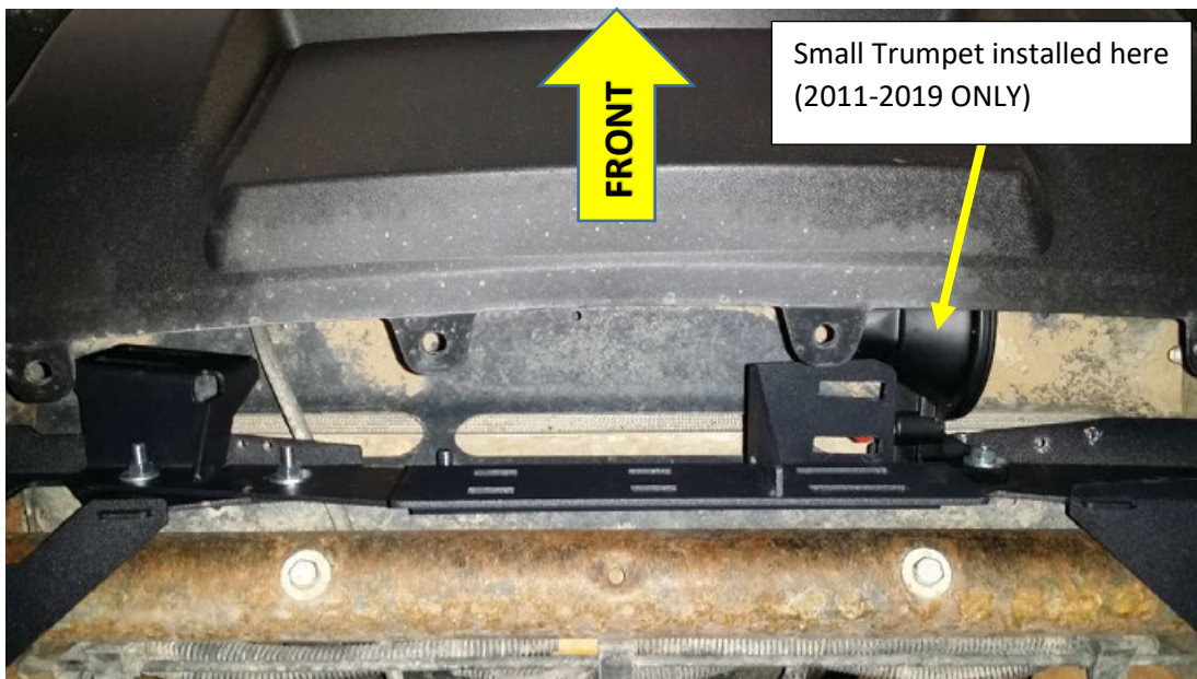
Figure 37 - HD18-303 Connector Bracket, installed
