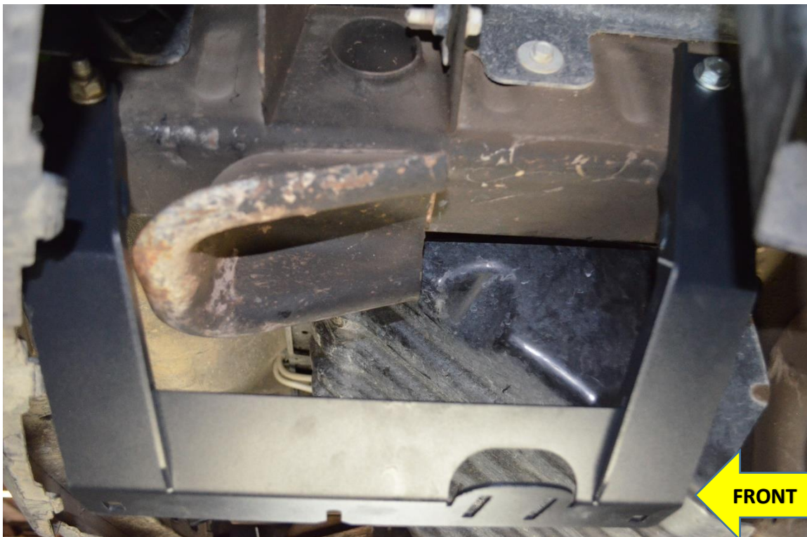
Figure 16 - Bracket Attached to Frame Rail (Driver Side)
