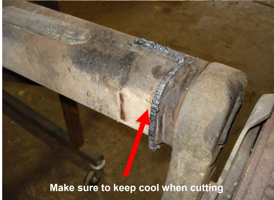
Old brackets cut off the axle
