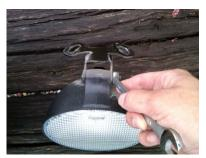
4. Reusing bracket, bolt, washer, and nut... reconstruct bracket assembly on new Model 735 LED lamp. Also use 2 additional new plastic spacer washers (included in upgrade kit). Assemble as per picture.
