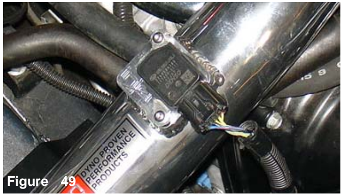
Figure 49 The electrical harness is firmly connected on the mass air flow sensor.
