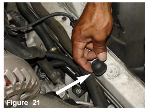
Figure 21 The rubber vibration mount is removed from the car frame as shown above. The new heatshield will be placed over the studs.
