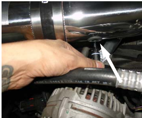
Connect the temperature sensor and install into the gromet from step 22.
