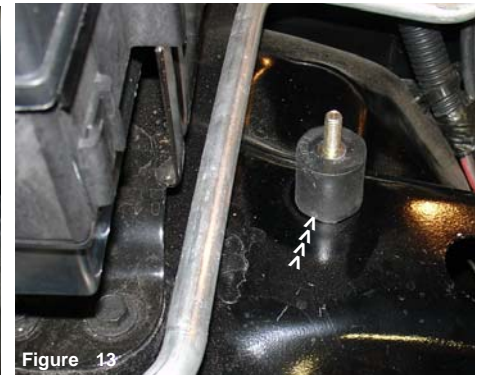
Figure 13 Using the fender washer and m6 flange nut the vibra-mount is now firmly in place.
