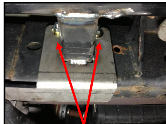
Figure 3 – U-Bolts Installed & Fastened
