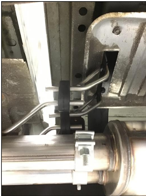
Figure 1 Before muffler hanger rod attachment to frame
