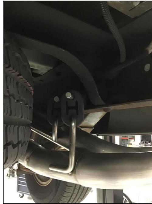
Figure 2 Rear tailpipe hanger to frame
