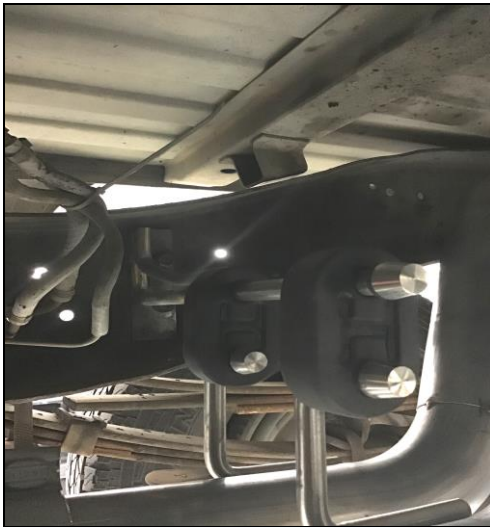
Figure 1 After muffler hanger rod attachment to frame
