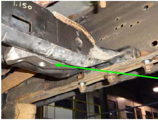
NEW RE-INDEXED TORSION BAR KEY BEING INSTALLED .
