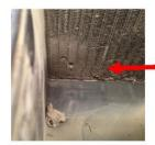
The deposited debris acts as an insulator to the thermistor probe; giving an incorrect reading.
