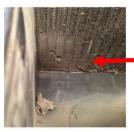
The deposited debris acts as an insulator to the thermistor probe; giving an incorrect reading.
