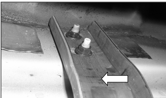
Shown the bracket installed.
