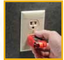
Test outlets protected by GFCIs
