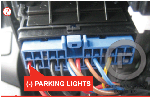
At parking light switch
