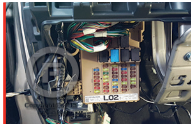
① ② ③ Fuse box.
