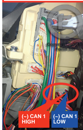
⑥ Behind Fuse Panel
