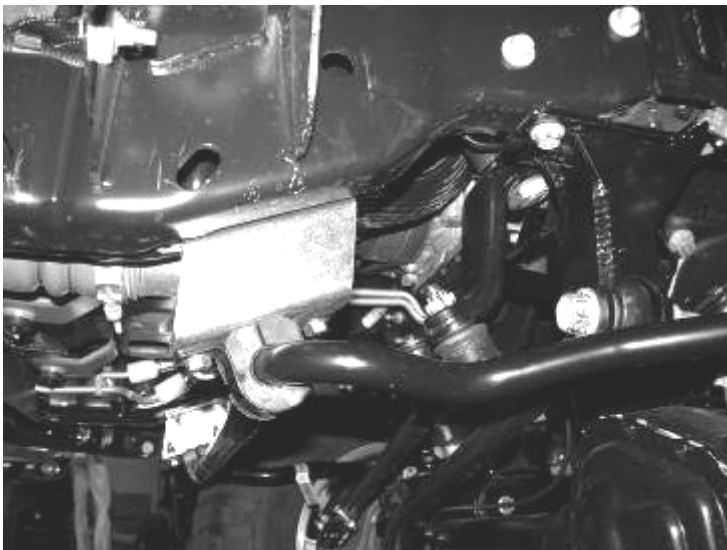
View of outer driver side frame rail
