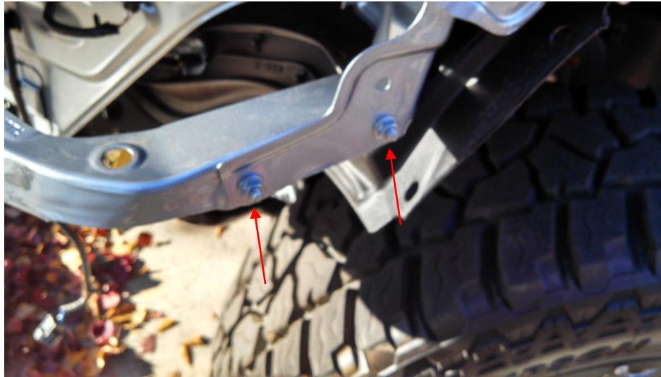
Figure 9 - Fascia Brace Nuts
