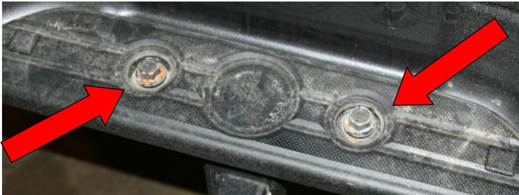
Figure 3 – Trailer hitch bolt removal
