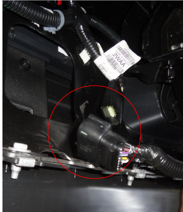
Figure 3(electrical harness disconnected)
