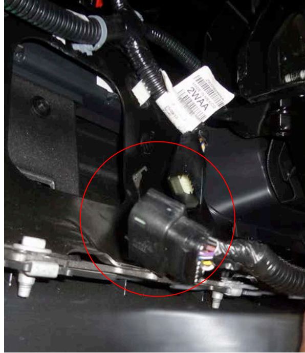
Figure 3(electrical harness disconnected)
