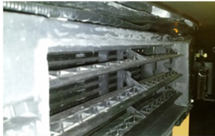
Figure 4 (Louver w/ shroud cut away at base)
