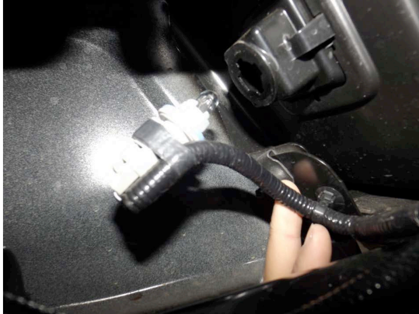
Figure 1 (Lic. Light removed)
