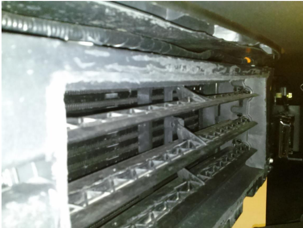
Figure 4 (Louver w/ shroud cut away at base)
